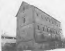
Fig. 14.232. Old building at the New Simonov Monastery in Moscow. General view. Photograph taken in 2000.
